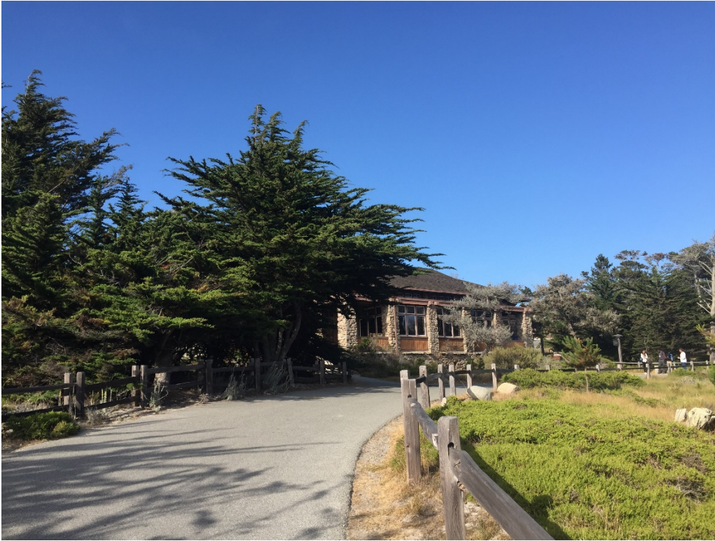
Main building used by the Society for Conservation GIS Conference at the Asilomar Conference Center in Monterey, California, United States
