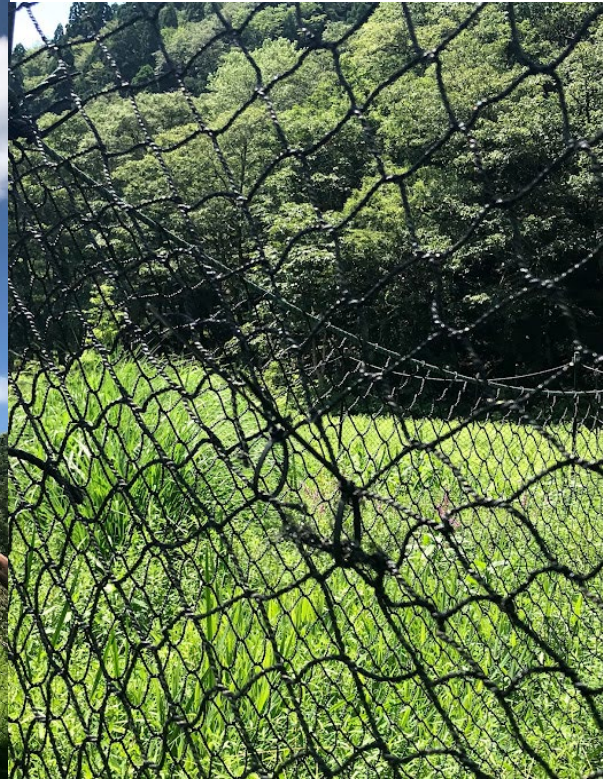
Fig. 8. Tightening the damaged holes to make it smaller
